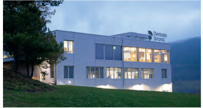
Our facility in Ballaigues, Switzerland uses 572 photovoltaic panels (930 m 2 ) implemented on the roof delivering 151.6 kWp.
